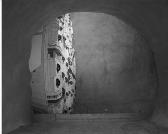
Fig. 11: Tunnel Amsteg, east tube, TBM cutter-head.
