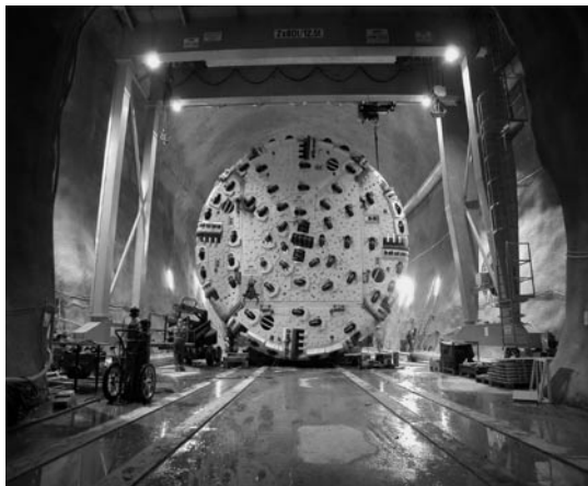
Fig. 12: Tunnel Bodio, installation of the TBM in an underground chamber.
