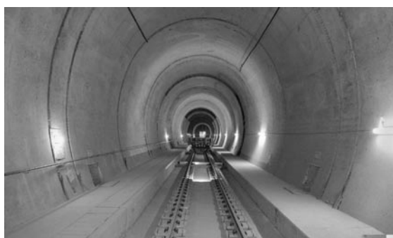
Fig. 8: Lötschberg Basis Tunnel, the inner lining will be finished soon.
