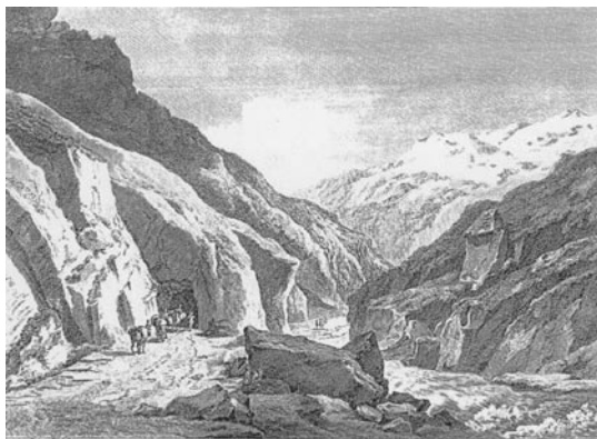
Fig. 1: The "Urnerloch", 1707, the first traffic tunnel in the Gotthard region.
