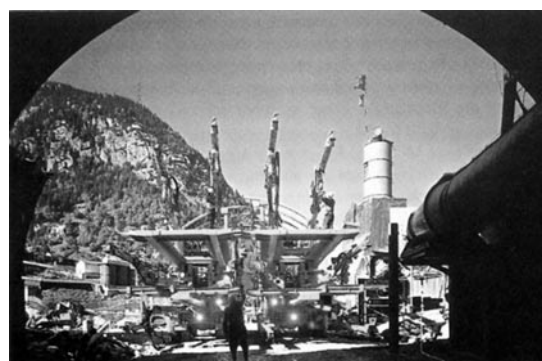
Fig. 4: Gotthard road tunnel; starting excavation in 1970.
